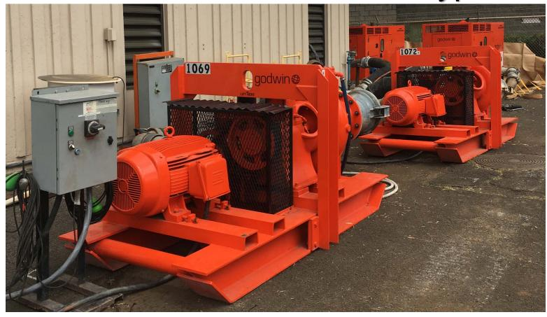
It is getting more and more common for our clients to be given permission to use station power for sewer bypassing and we are embracing it! Pacific Pump & Power has been adding more electric powered equipment to our fleet to complement the diesel units.
